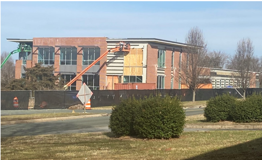
Construction of the Woodrow W. Bolick Center. Photography by William McAuliffe
